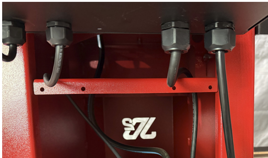
Figure 7.1: Route the motor and valve cables.
